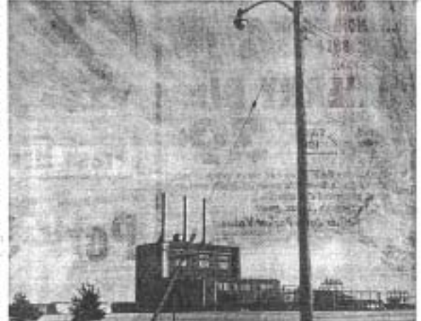
SOURCE OF POWER AND REVENUE — The Hamilton Justice R. Wolkstein generating plant of the Consumers Power Co. is at the south end of the proposed Luna Pier incorporation area. Supplying electricity to southeast Monroe County, the plant also would provide a solid tax base for the proposed City of Luna Pier.
